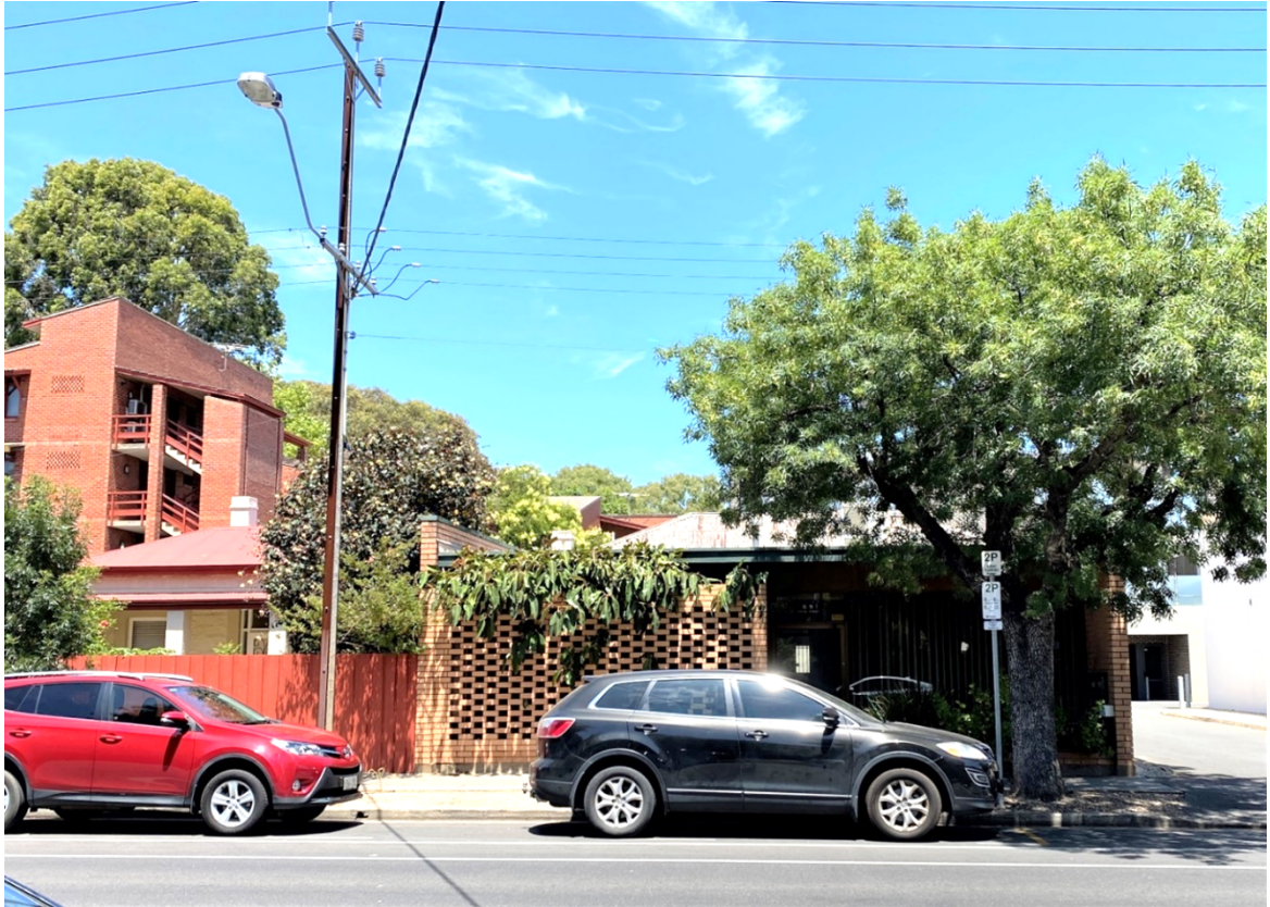
Photo 3.1 – existing building viewed from Finnis Street
