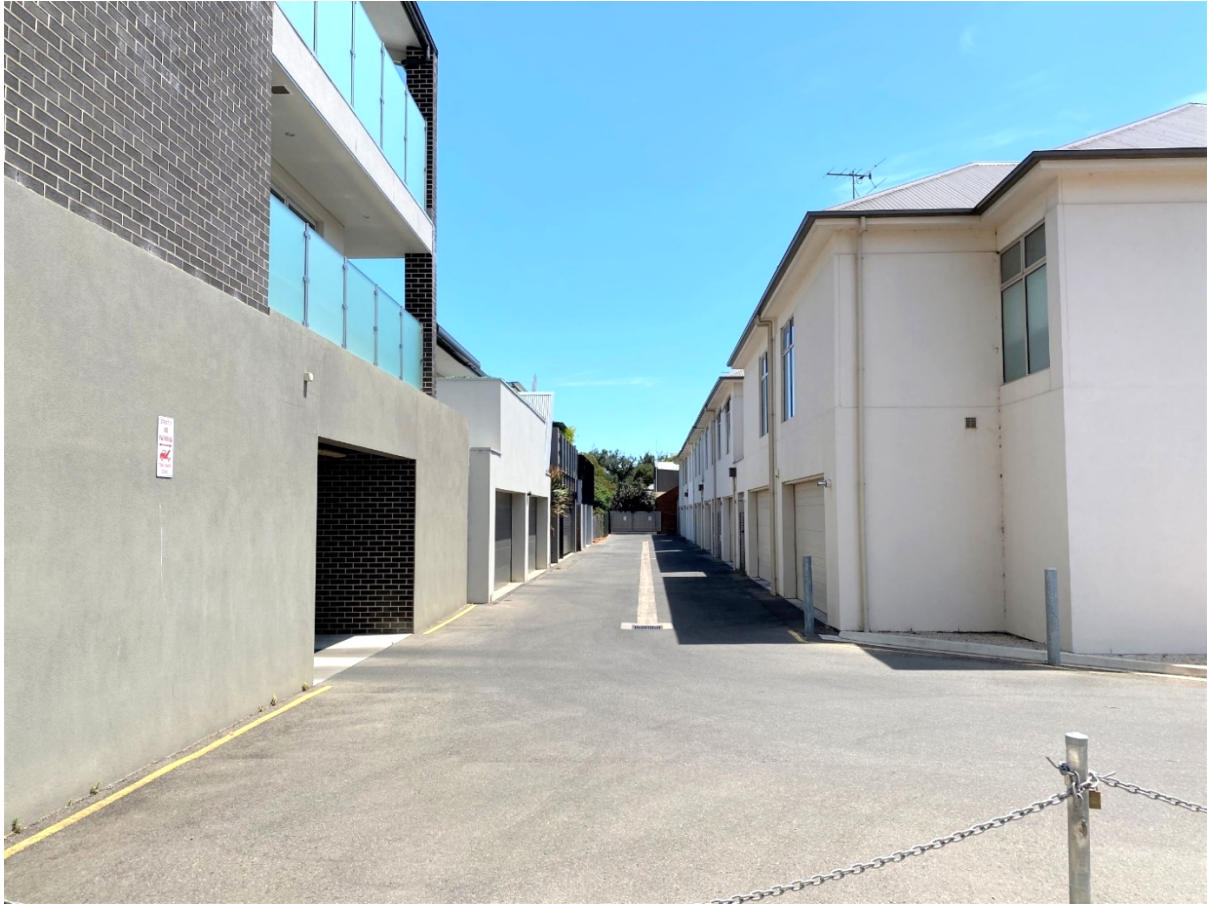
Photo 3.7 – view of right of way to the west
